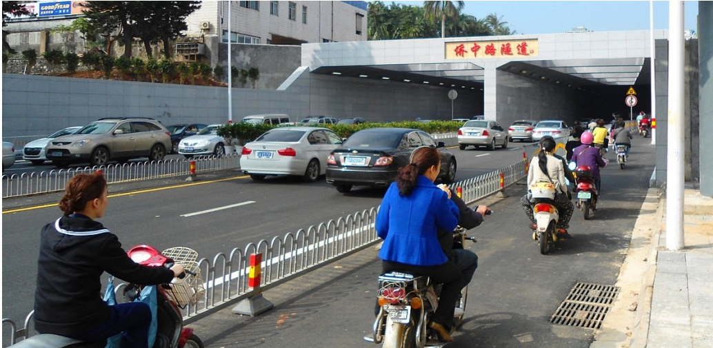
Figure 4: Qiaozhong Road tunnel (Wikiwand.,n.d.)
