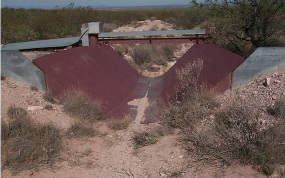
Figure L.3.16. Santa Rita supercritical flume installed in the outlet of the Tromble Weir watershed (Credit: Turnbull et al., 2013).
