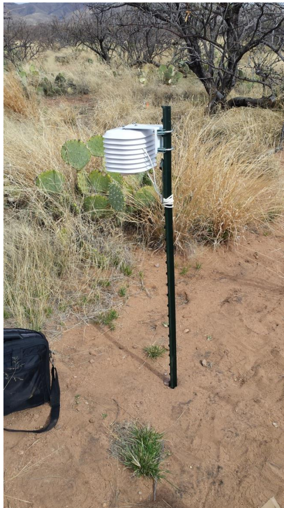
Figure K.1.2. Air temperature and relative humidity sensors installed in the field site, including the solar radiation shield.
