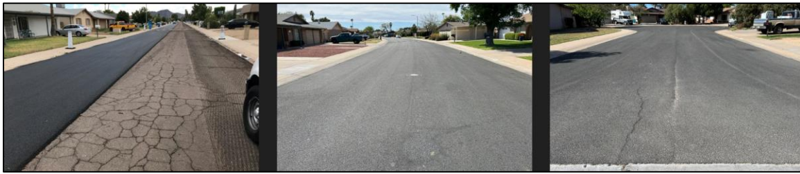
Figure 7-15: Pavement Condition Before, During, and After UTBWC Treatment in QS 30-20
