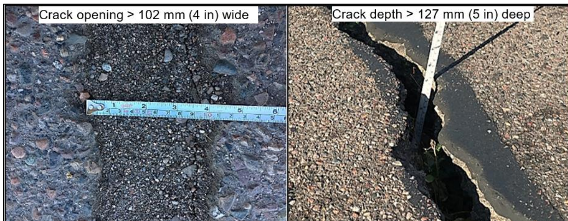
Figure 7-9: Transverse Cracking
