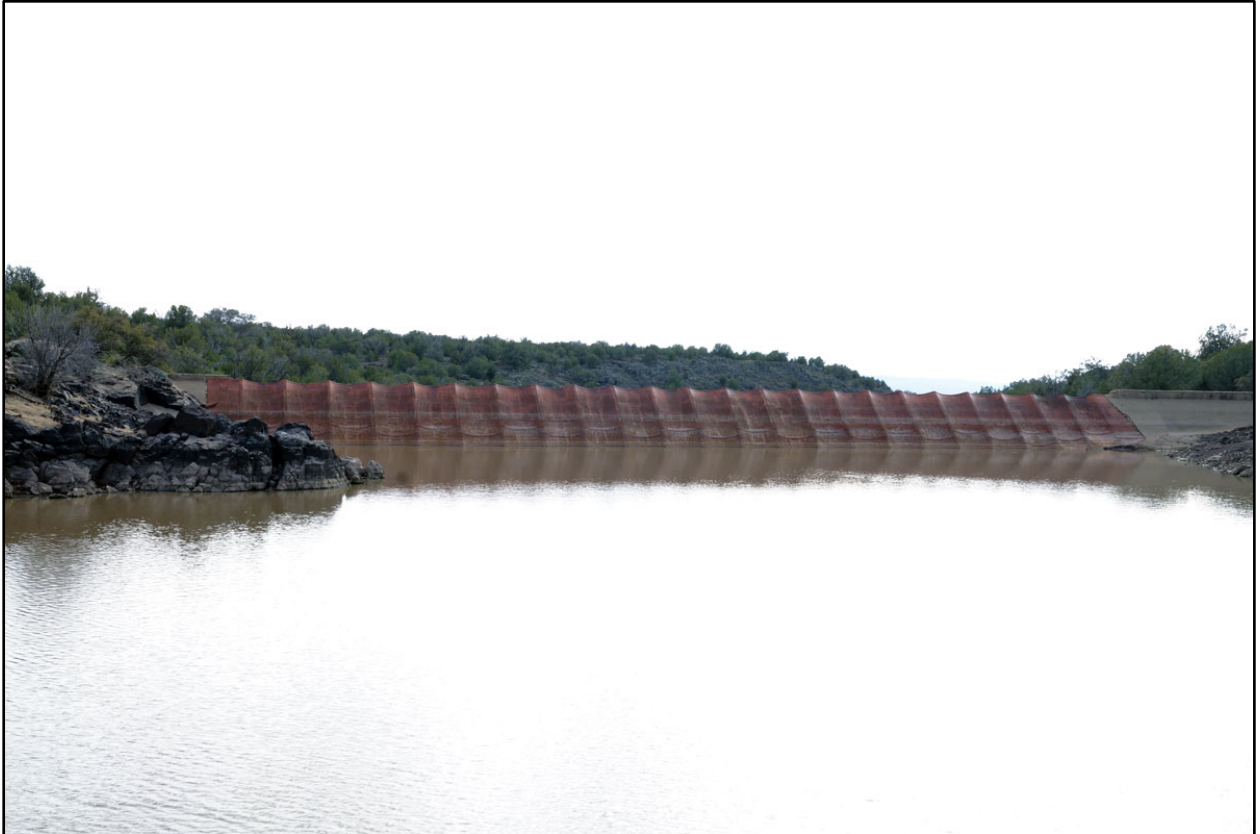
Figure 10. Known today as Bainbridge Steel Dam, the dam designed by F.H. Bainbridge is one of only two remaining steel dams in the world. Shown here from behind, the large reservoir is visible with the top of the steel dam visible in the background. The concrete abutments built into the bedrock are visible on either side. The Santa Fe Railroad called the dam simply Dam No.1. Photograph: Daniel Milowski, Bainbridge Steel Dam, 2020. Author's personal collection, Tempe, AZ.
