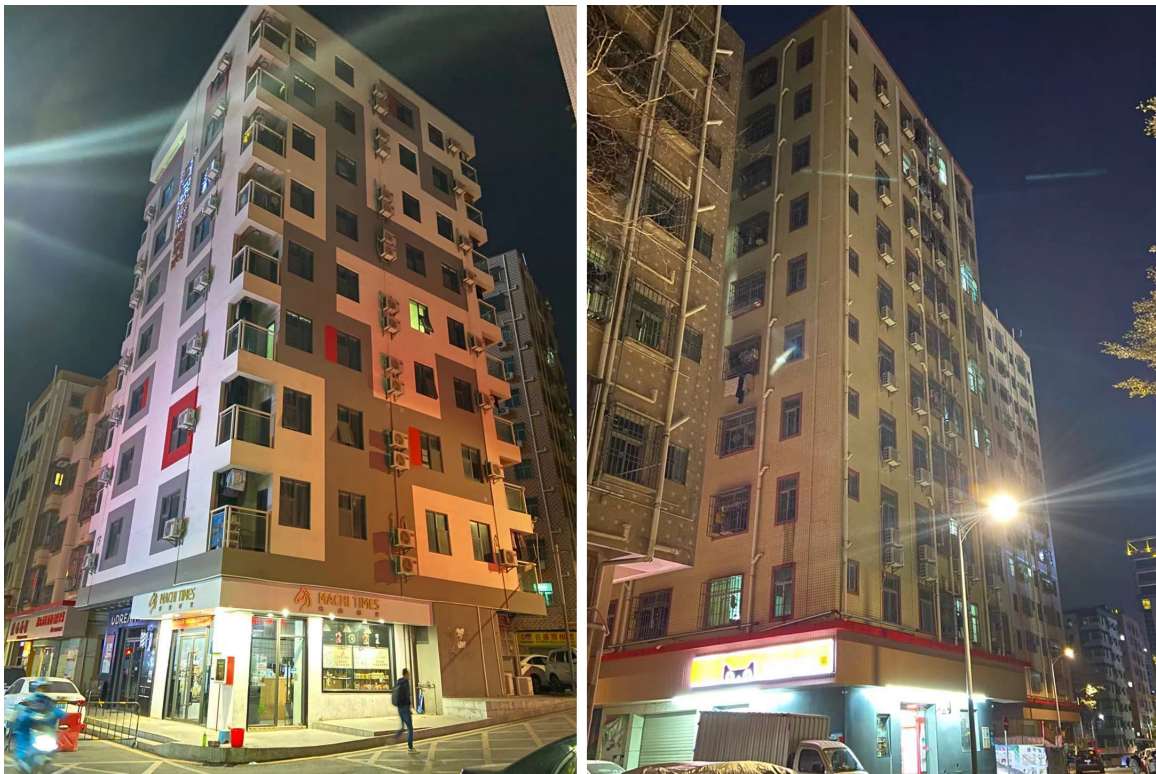
Figure 8.2: Vanke Renovated Apartment (left) and Villager Housing (Right) 11
