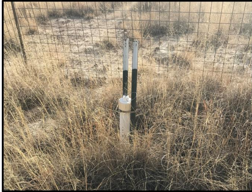
Figure F2. Water level sensor at Playa 17, representative of how the sensors are installed at all playas.
