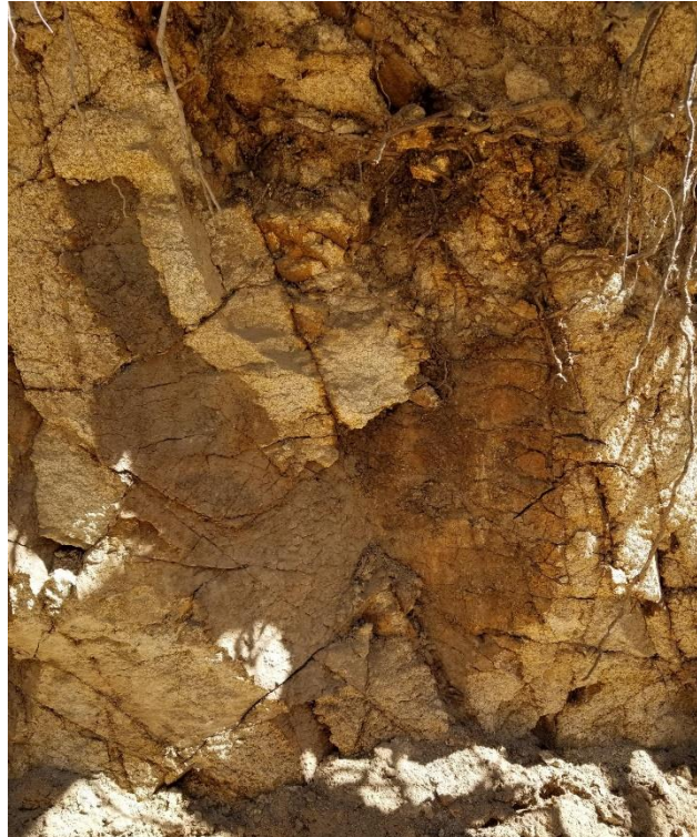
Figure 3- Typical coloration and coating on joint surfaces.
