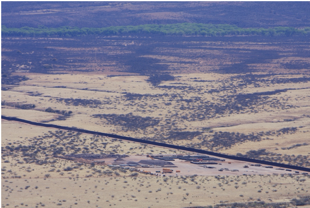
Figure 14. Border wall and construction staging area seen from nearby mountain
