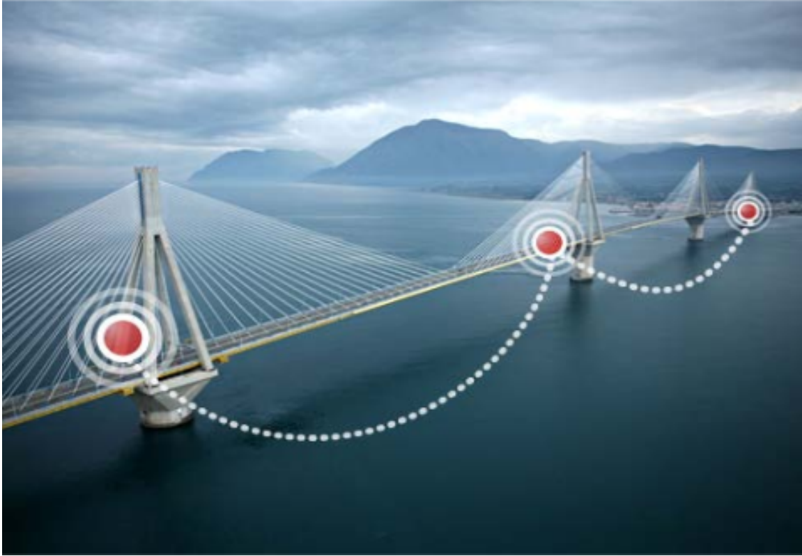
Figure 24. Structural Monitoring of Bridges
