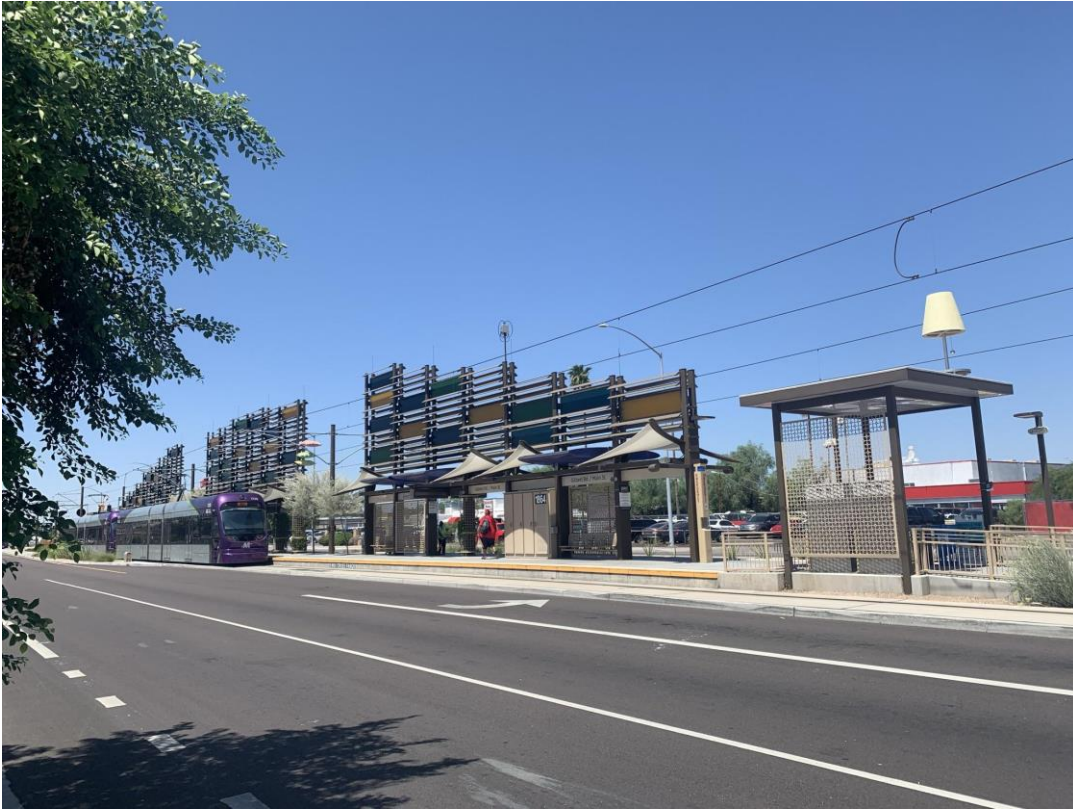
Figure 11 - Gilbert/Main St Station
