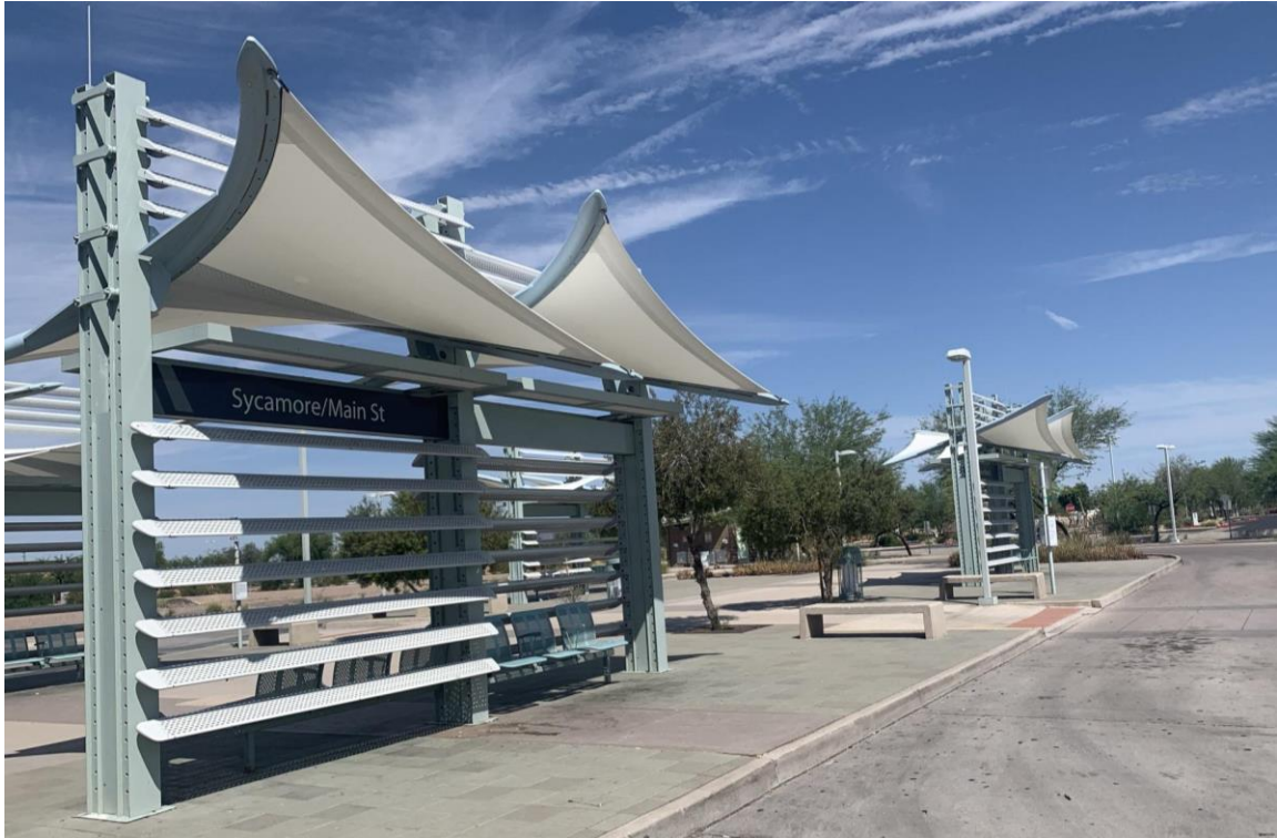
Figure 15 - Sycamore/Main St Station, transit center's bus stops
