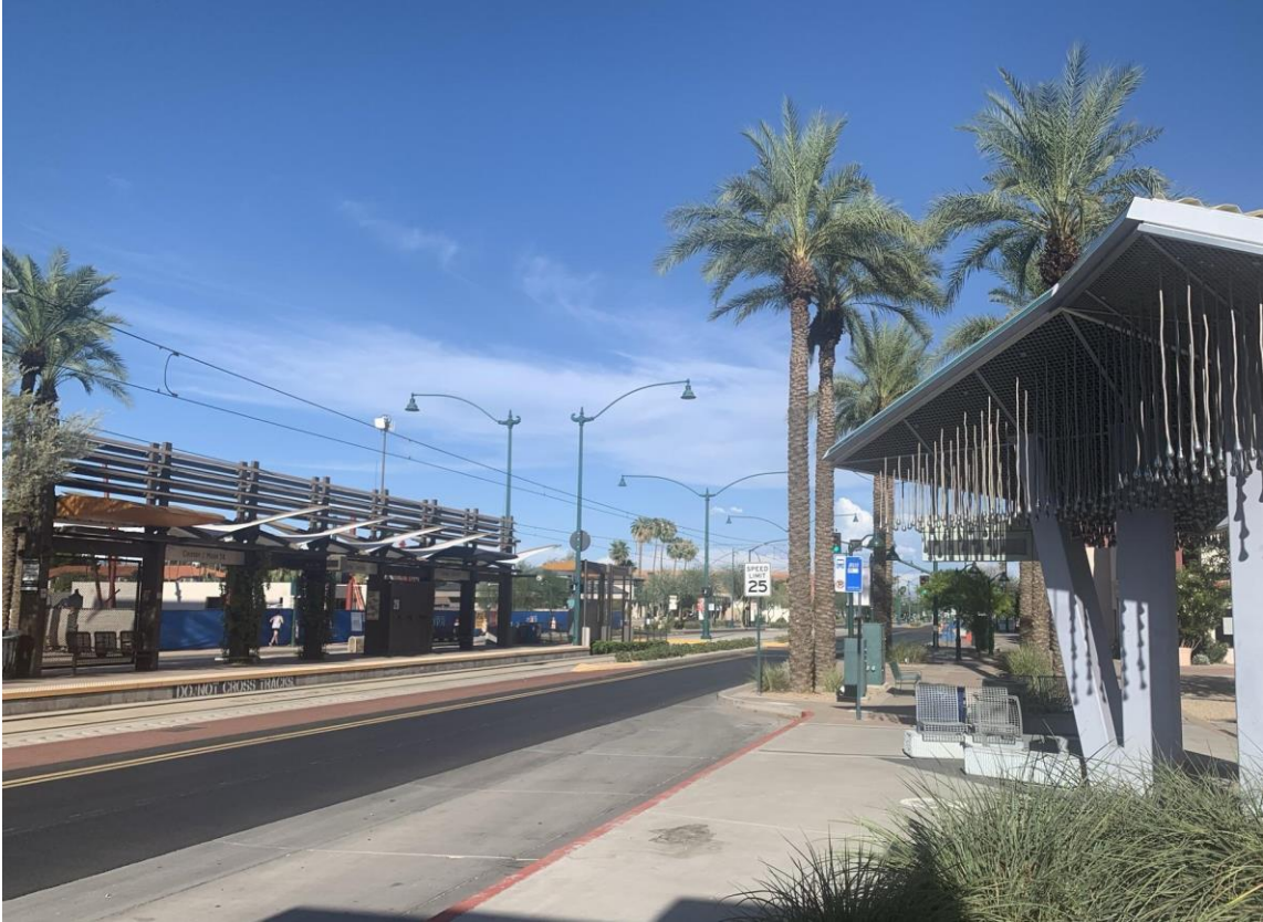
Figure 13 - Center/Main St Station
