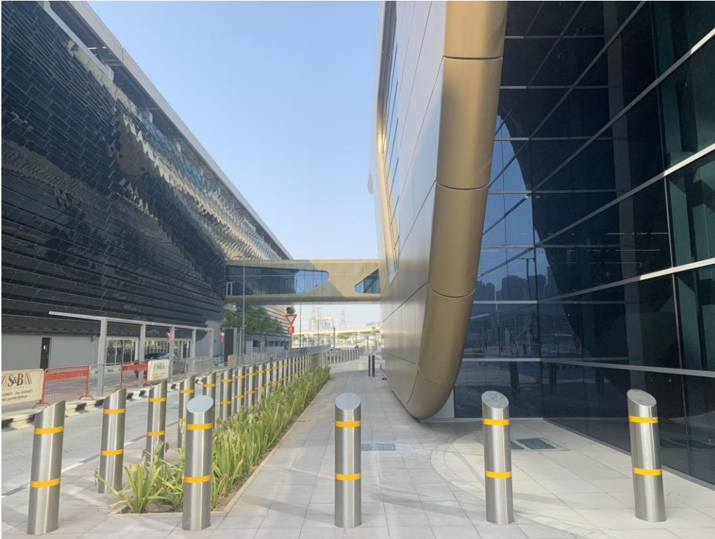
Figure 3 - Jebel Ali Station (right) and parking structure (left)
