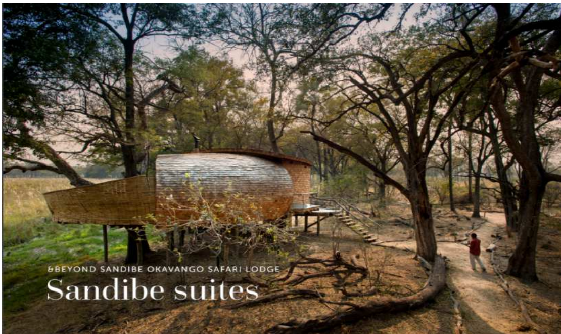
Figure 4.6: Sandibe Okavango Safari Lodge Suet Section (Sandibe Okavango Safari Lodge / Nicholas Plewman Architects in Association with Michaelis Boyd Associates | ArchDaily, n.d.)
