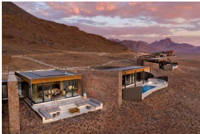
Figure 4.14: Sossusvlei Desert Lodge PV Panels (AndBeyond Sossusvlei Desert Lodge / Fox Browne Creative, Jack Alexander | ArchDaily, n.d.)
