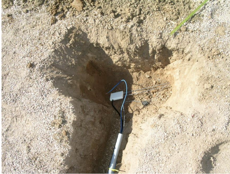
Figure 3: Installation of CS616 soil moisture sensor at xeric site.
