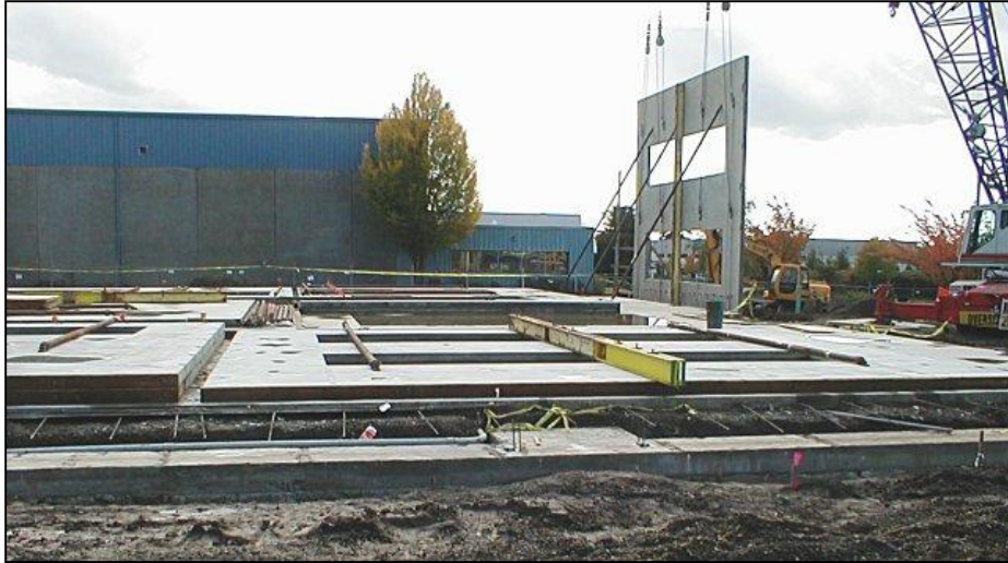
Figure 9: A Tilt-Up concrete construction at site. (Source: Wikipedia)
