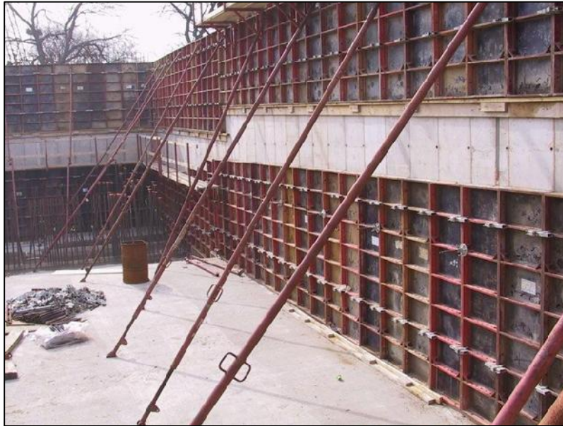
Figure 10: Framework for Precast concrete wall (Source: Baruzzini Construction)
