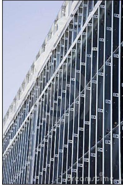
Figure 15: Steel Stud Wall of an Industrial Building (Source: Dreamstime)
