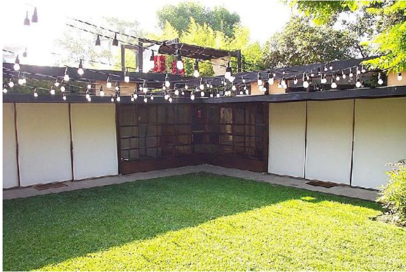
Figure 8: Schindler-Chase house (Rudolf Schindler) is an early example of Tilt-Up concrete construction
