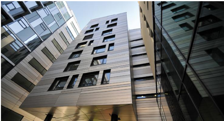
Figure 12: Metal Facade Panel Location: Bratislava Slovakia (Slovak Republic) (Source: Hunter Douglas Facade systems)
