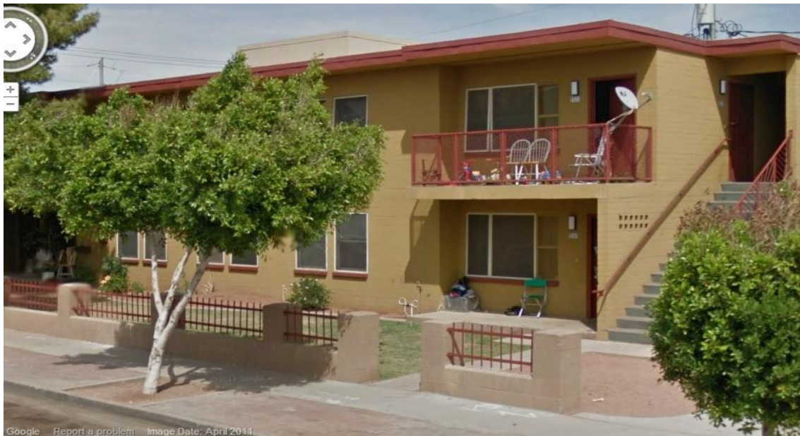
Figure 13. Two-storied block consisting of six units each, un-insulated concrete blocks
