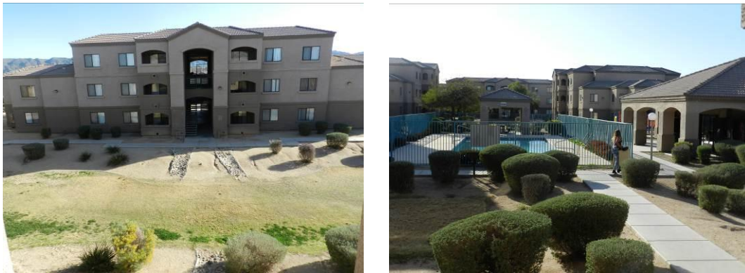
Figure 13. Vineyard Estates: swimming pool, ramada and property office (on the right), one of the buildings (on the left) (March 2013)
