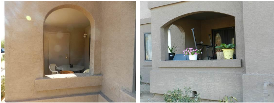
Figure 16. Seating places on balconies in Vineyard Estates (March 2013)
