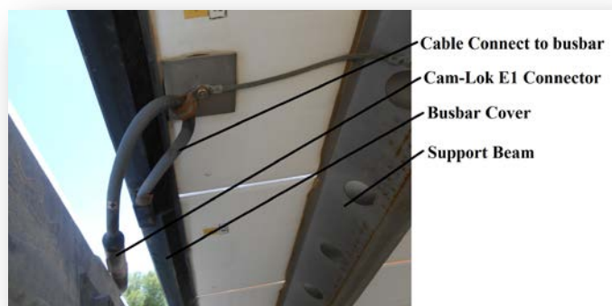
Figure 23 – Cable Interconnections Between Panel Groups
