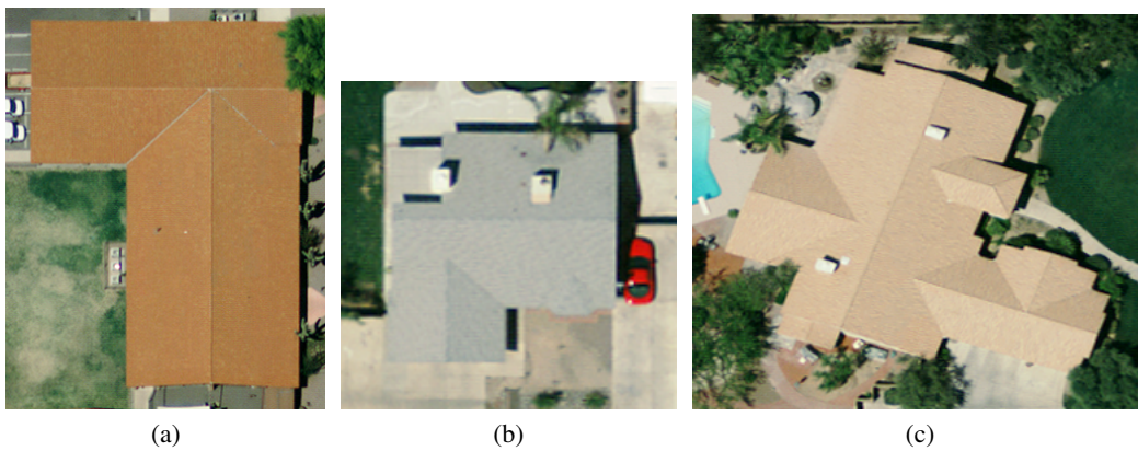
Figure 3.9: Different challenging gable interactions; (a) shows a roof with two pieces meeting at the ridge of gable; (b), (c) show roofs where individual pieces don't meet exactly at the gable ridge of each other
