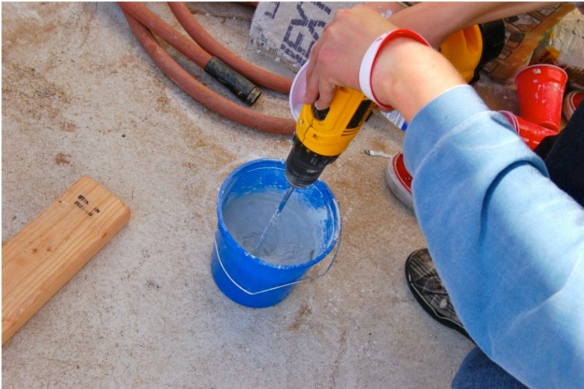
Figure 23. Mixing the grout using the cordless drill and paddle mixing attachment
