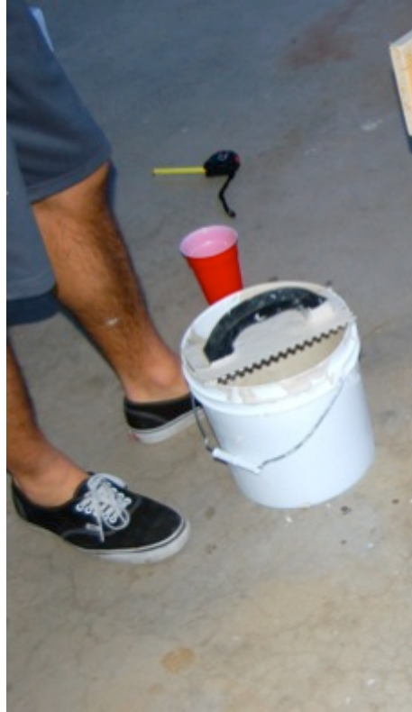
Figure 19. Bucket of mixed thinset with \frac{1}{4} " notched trowel
