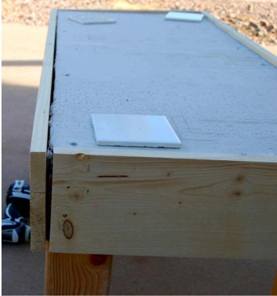
Figure 18. Trim Boards bowed out due to cement and plywood cut to large
