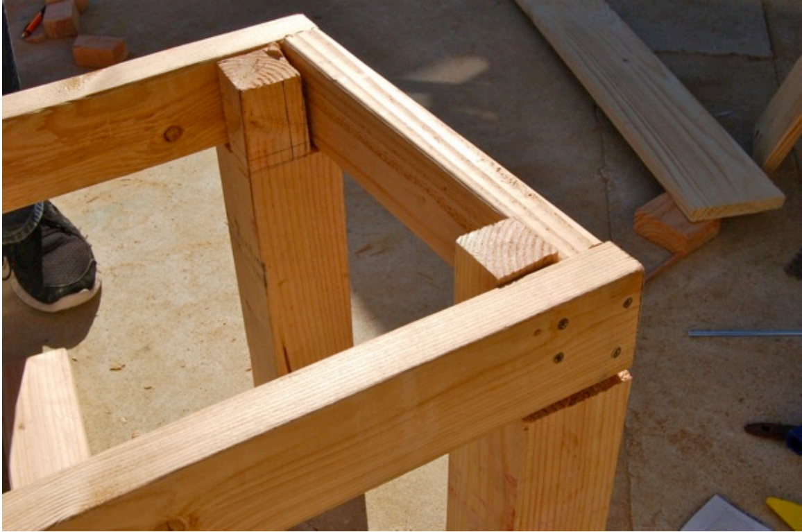
Figure 14. Joints misaligned during assembly due to poor craftsmanship in Phase I
