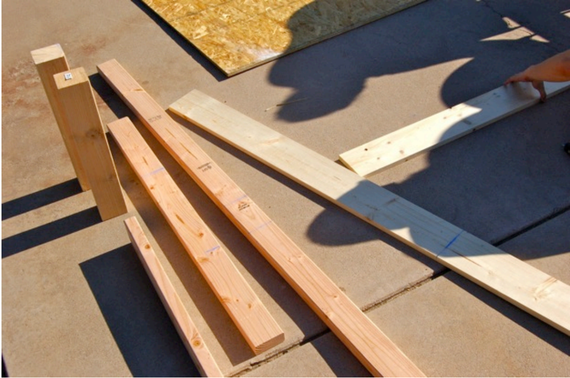
Figure 10. Wood was marked by one team using a chalk line
