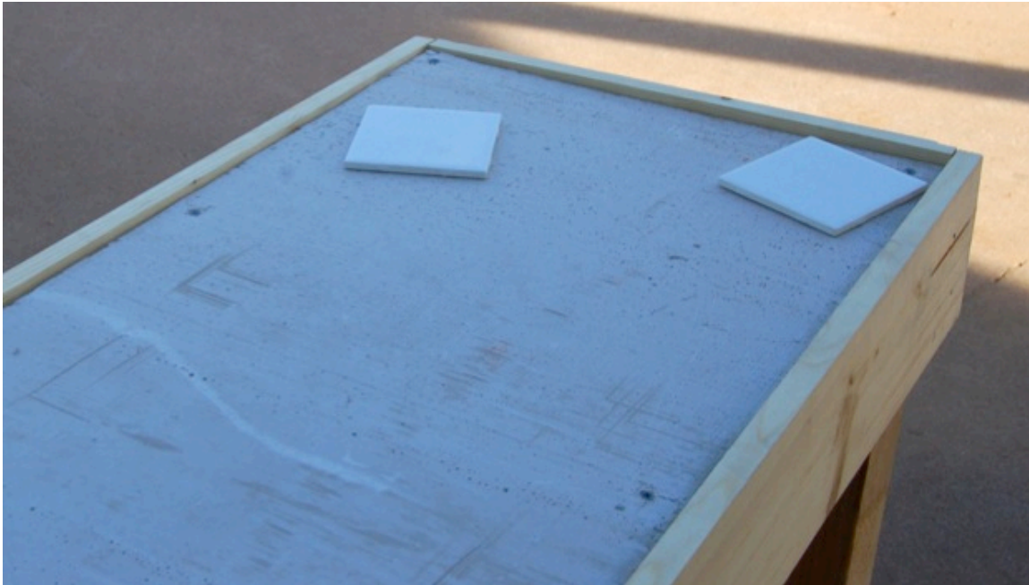
Figure 16. Tiles used as spacers to gauge trim height
