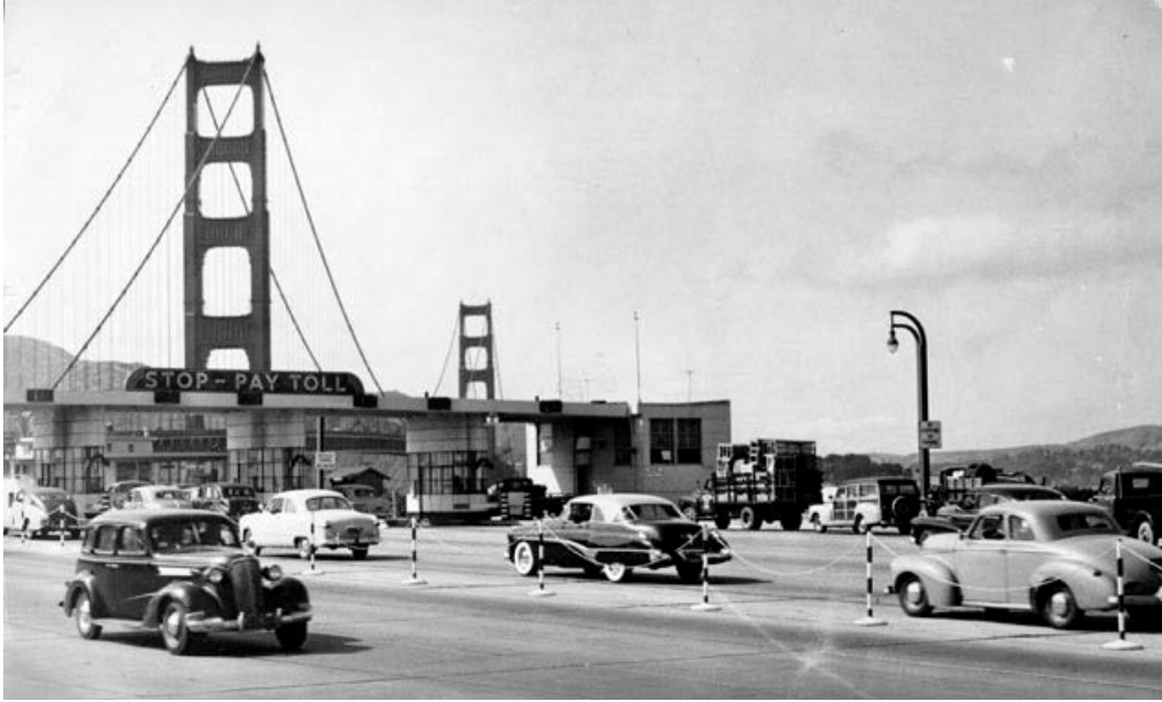
Figure 18 Presidio Parkway then known as Doyle Drive late 1930's (Arup/Parsons Brinkerhoff 2010)
