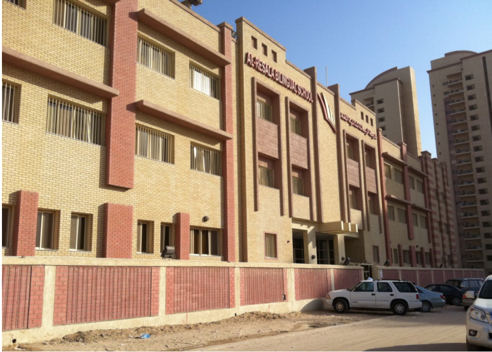
Figure 67. The side façade of the school.
