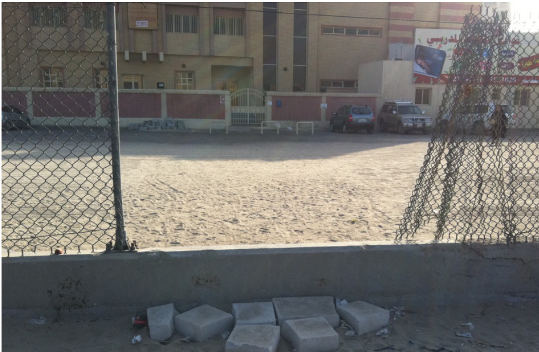
Figure 64. The wire gate, broken to ease the entrance to the school.
