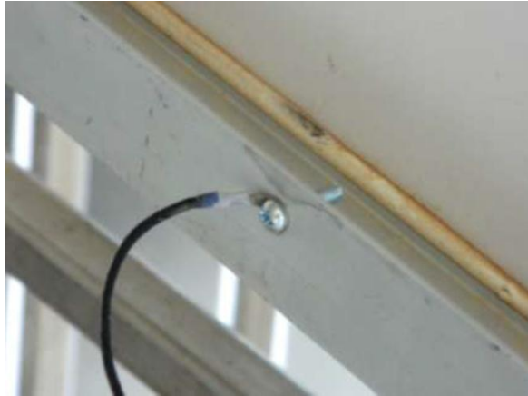
Figure 3.17: Positive from the power supply is connected to the grounding point.
