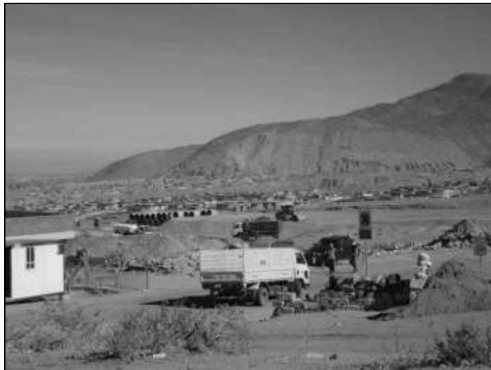
Figure 12: Potable Water Treatment Plant Construction Site. Photography by Author taken July, 2010
