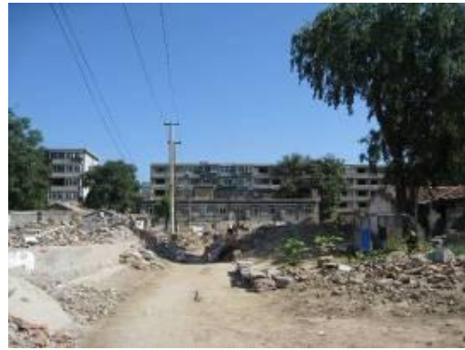
Land clearance underway
