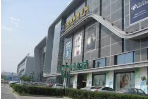
Commercial Cluster A Longde Square: Wanda International Cinema & Cuiwei Department Store
