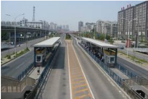
Exclusive Lanes for BRT Line 3
