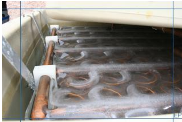
Figure 2.6 Ice Bear thermal storage [13]
