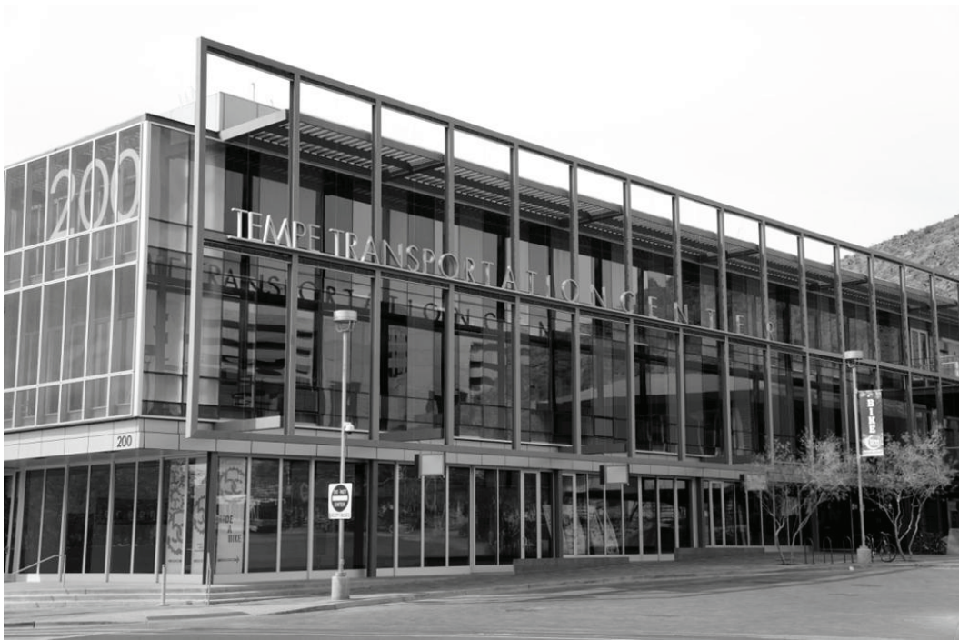
Figure 2. Transportation Center Building, Southeast view.
