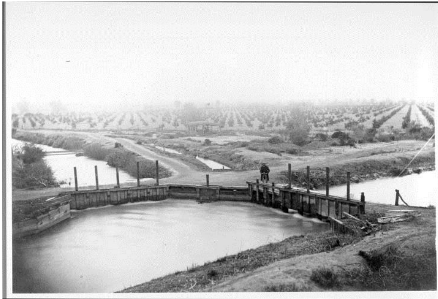
Figure 5 Main Gates of Crosscut Canal 1890 120
