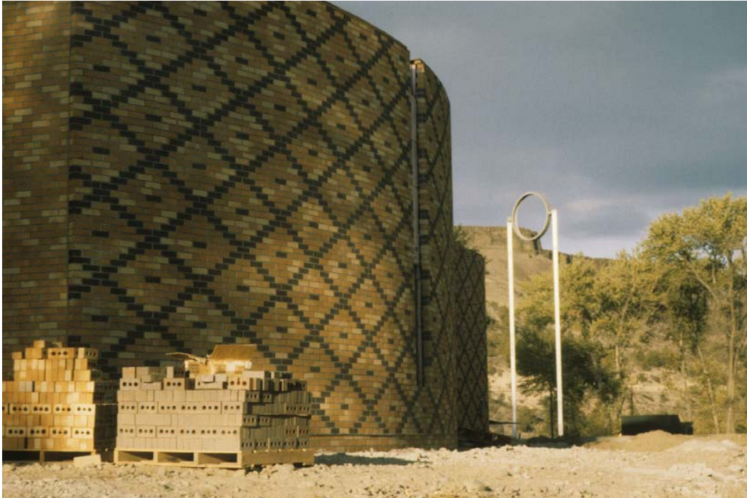
Figure 5.5. Patterned brick. Courtesy of Stastny Brun Architects from the Stastny and Burke project archives.
