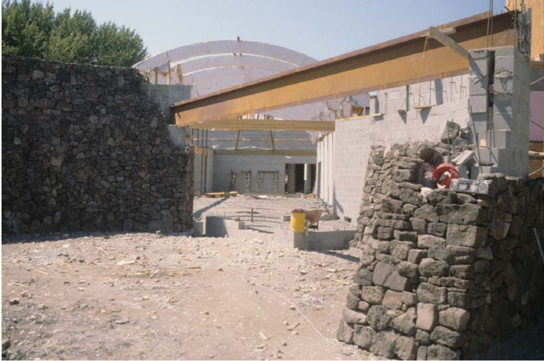
Figure 6.18. Entry drum with beam to support stone sign with curved glulams over lobby behind. Courtesy of Stastny Brun Architects from the Stastny and Burke project archives.
