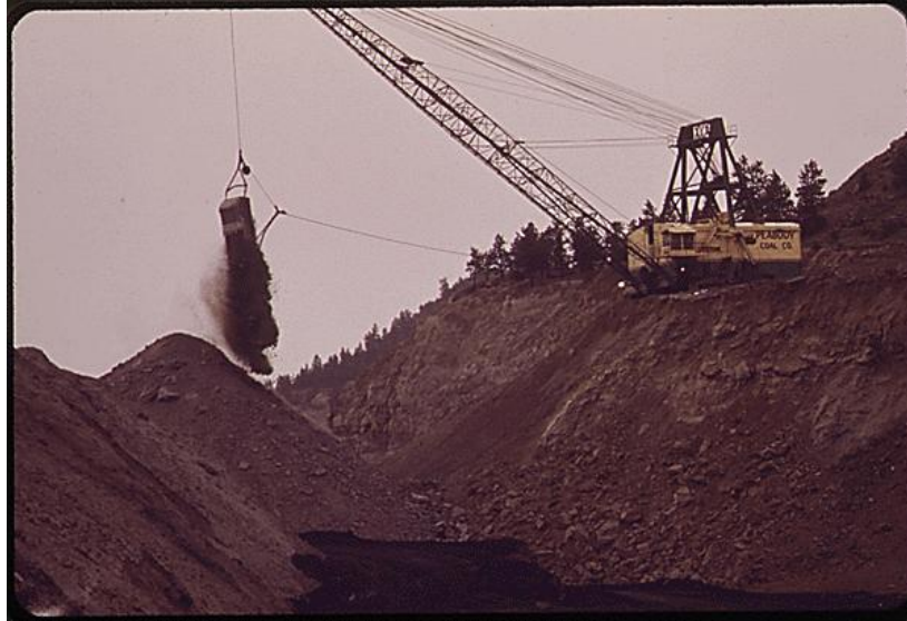
Photograph No. 549126 (Photographer Norton Boyd); “Peabody Coal Company strip mine, south of Colstrip, 06/1973,” June 1973; Documerica Project, Records of the Environmental Protection Agency, 1944-1006, Record Group 412; [Online version, www.archives.gov , National Archives and Records Administration, 5 December 2011], National Archives at College Park, College Park, MD.
