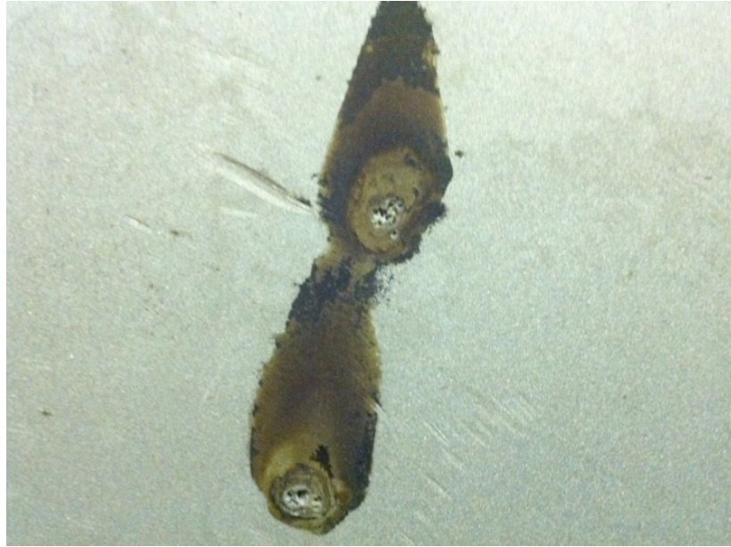
Figure 2.2 Magnified Image of Pitting and Stress Corrosion Cracking
