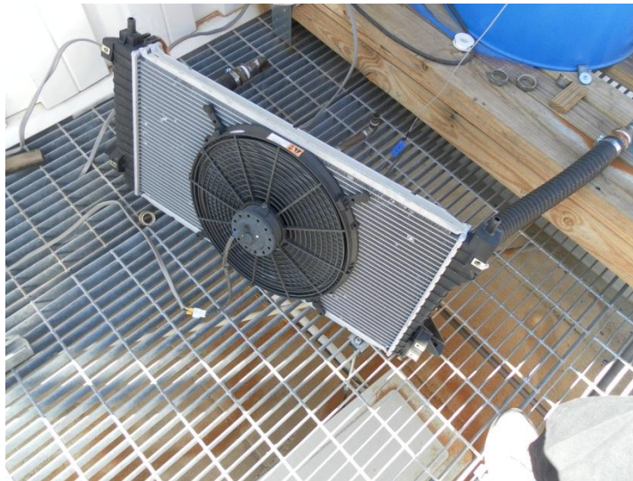
Figure 17. Heat dump for the collector array
