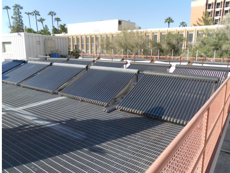
Figure 14. Apricus AP-30 collector array
