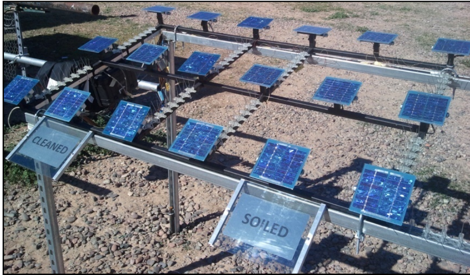
Figure 3.4 System Array in the field
