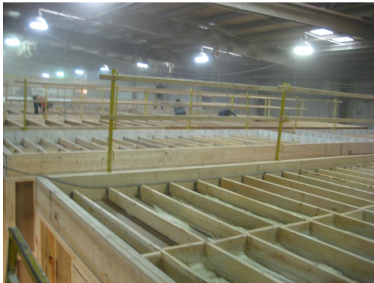
Figure 14. Module ceilings ready for insulation and roof installation.
