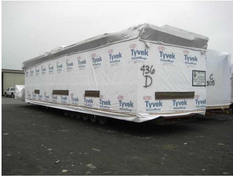
Figure 22. Module shown with house wrap protection being readied.
