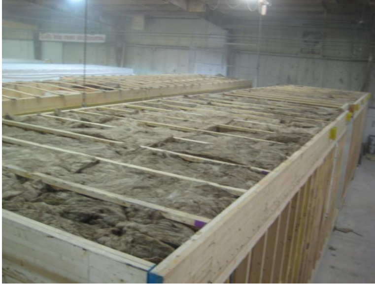
Figure 15. A module ceiling after insulation has been added.
