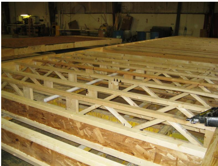
Figure 7. Web-style floor trusses used in flooring for plumbing access.
