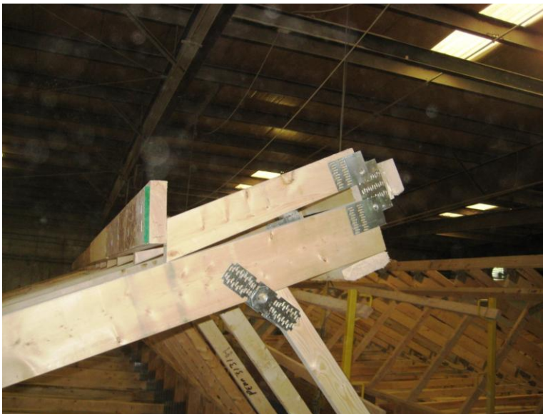
Figure 16. Module roof showing close-up of hinged component.
