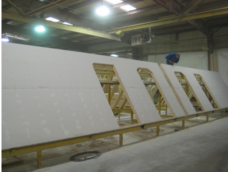
Figure 10. Completed exterior wall with drywall installed on inclined framing table.
