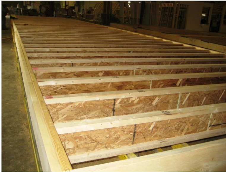
Figure 6. Fabricate I-joist floor trusses.
