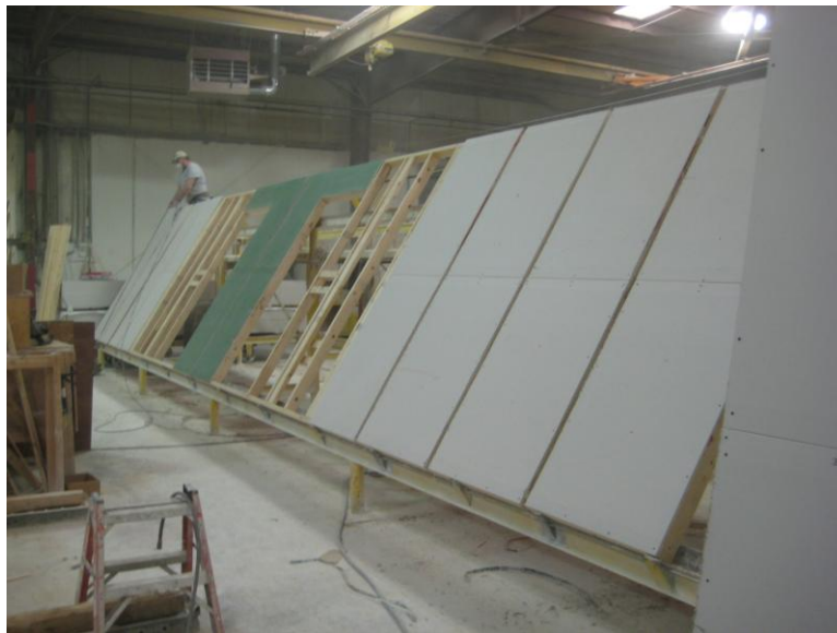
Figure 12. Drywall applied to framed exterior wall on inclined framing table.
