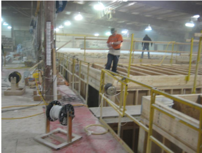
Figure 13. Workers installing module ceilings.
