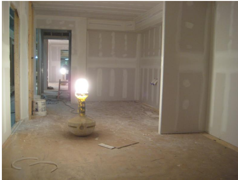
Figure 18. Interior of module showing drywall finishing.
