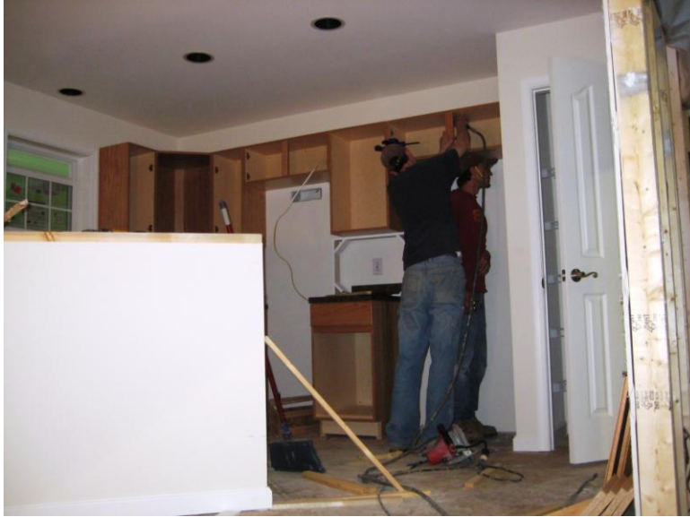
Figure 20. Cabinets being installed in the modular home.
