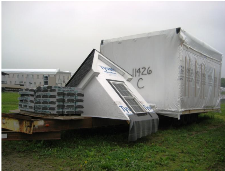
Figure 23. Completed module ready to be delivered.
