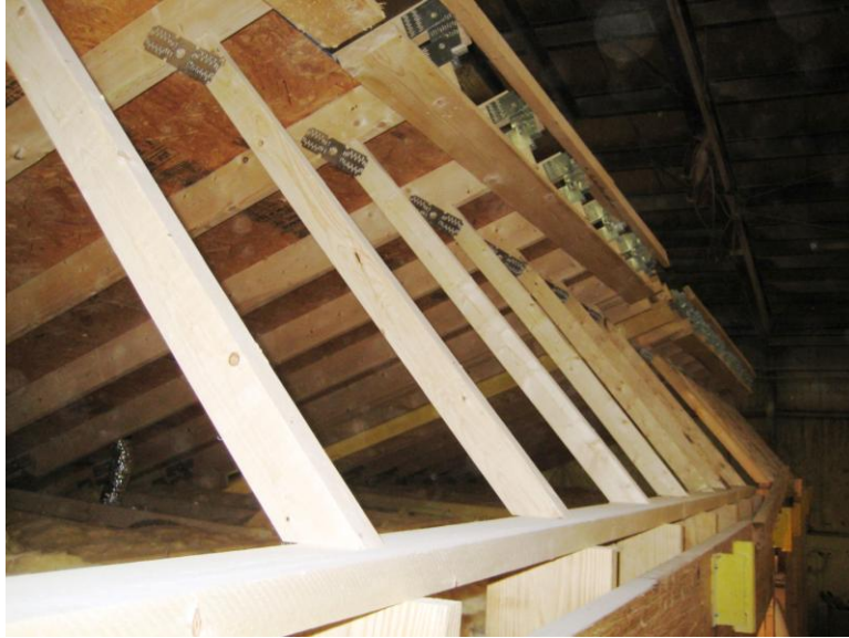
Figure 17. Module roof showing wall bracing.
