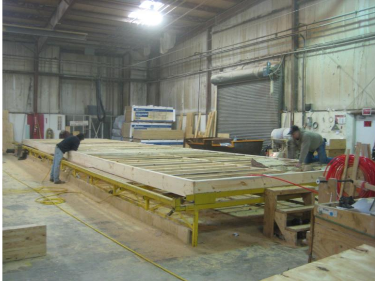
Figure 8. Workers building floors on floor jig using dimensional lumber.
