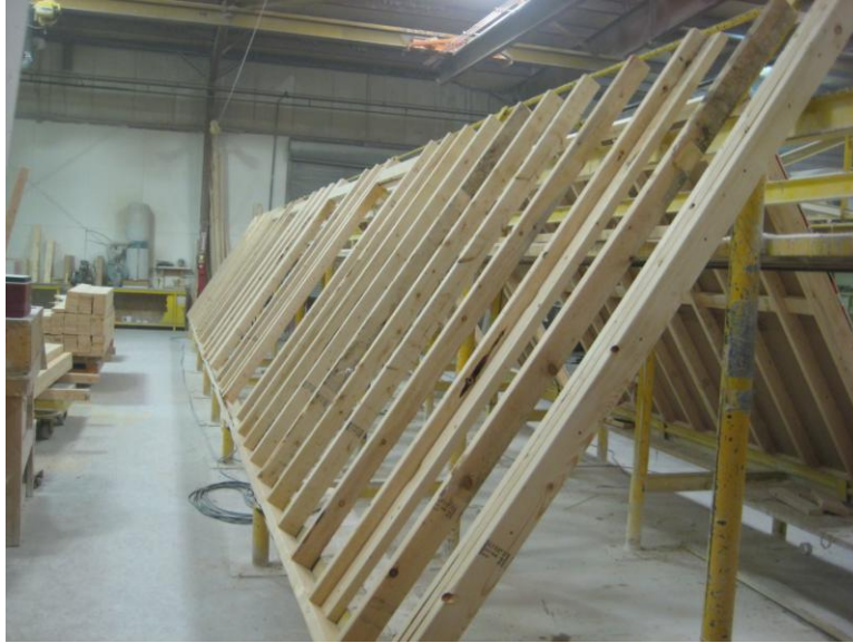
Figure 11. Exterior wall framed with dimensional lumber on inclined framing table.
