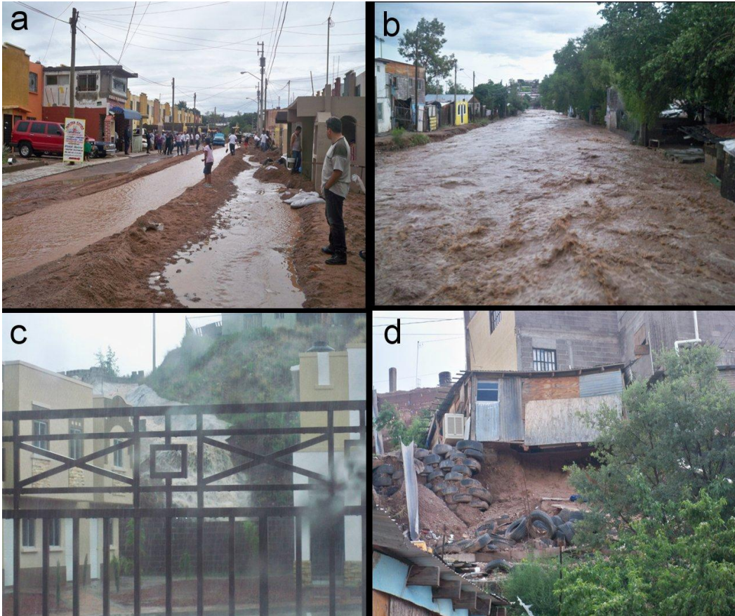
Figure 11. Flooding in Ambos Nogales, July 2010 (a) Middle-income neighborhood affected by flood. (b) Urban river (c) Runoff going through high income neighborhoods. (d) House with a foundation of tires. (Source: Protección Civil )
