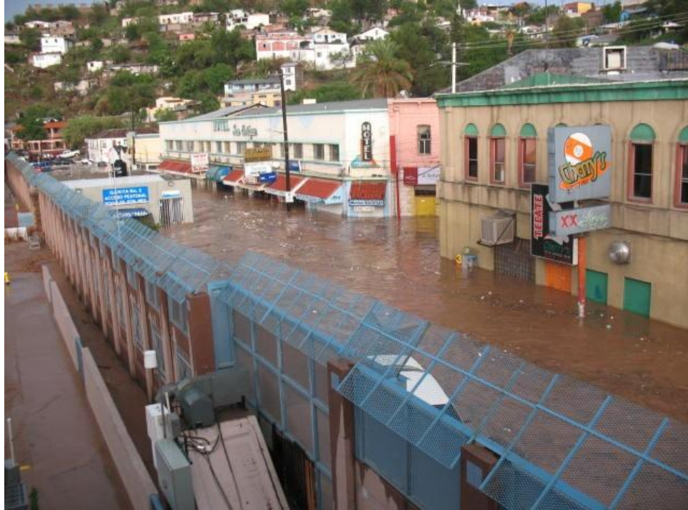
Figure 25. Unintended dam created by the border wall during the flood of July 2008 in Ambos Nogales. (Photo provided by City Planning, Nogales, Arizona)
