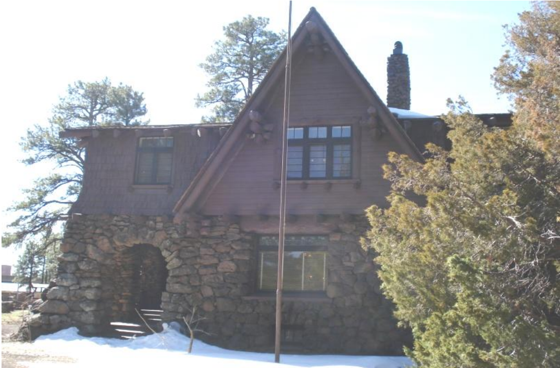
Figure 12. North side of East House. Photograph by author, 2009.
