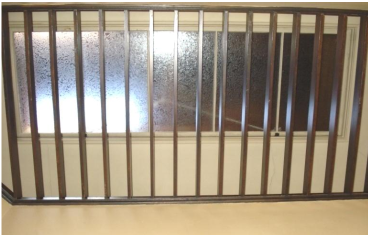
Figure 75. Light Well: East House, first floor view. Photograph by author, 2009.
