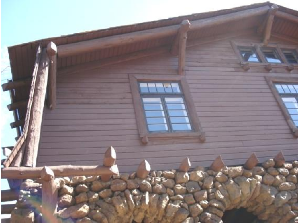
Figure 15. West House, Joinery and roof detail image. Photograph by author, 2009.
