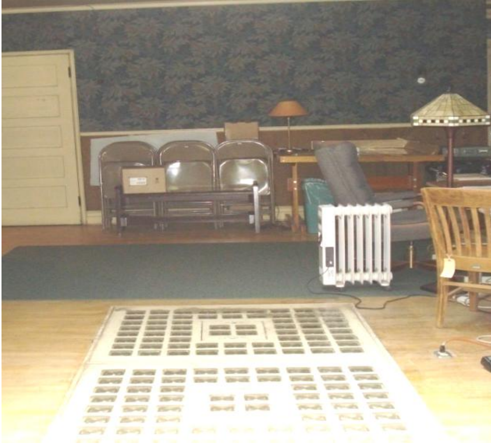
Figure 73. Light Well, second floor view: West House. Photograph by author, 2009.
