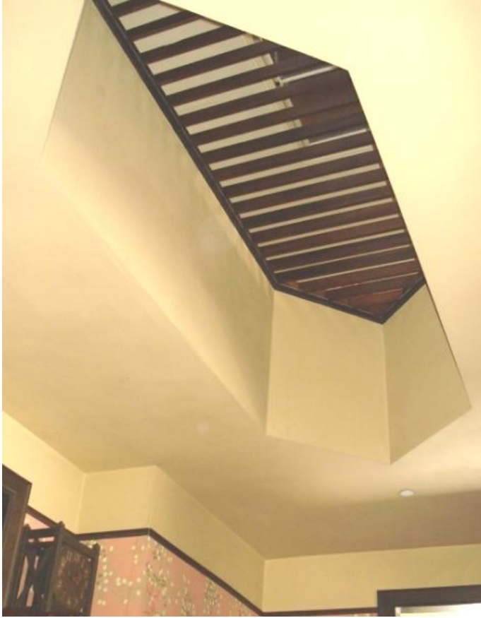
Figure 74. Light Well: East House, first floor view. Photograph by author, 2009.
