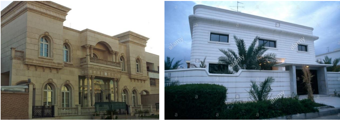
Figure 7 Typical villas in Kuwait
