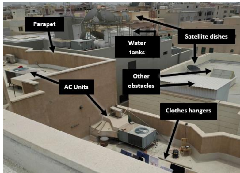
Figure 28 Rooftop image showing typical flat roof and layout of obstacles
