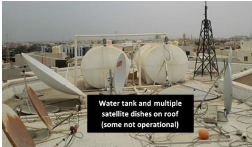
Figure 29 Image showing random placement of objects on roof occupying usable solar area
