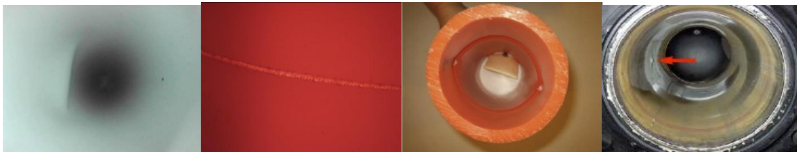
Figure 3-2. Four types of common damage in pipe: dent, slit, squeeze-off and impingement (from left to right)
