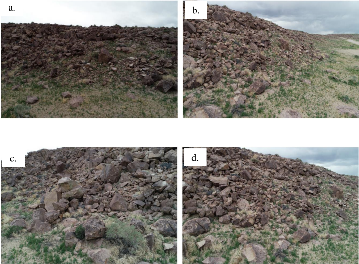
Figure 4. Field photographs of a normal fault scarp (in the C3 survey) that is approximately 5-12m high. Commonly observed is a more resistant upper face transitioning to a moderately sloping mid scarp strewn with poorly sorted angular particles ranging in diameter from centimeters to two meters. The lower slope is subdued due to an influx of windblown dust. Photo locations in Figure 7.
