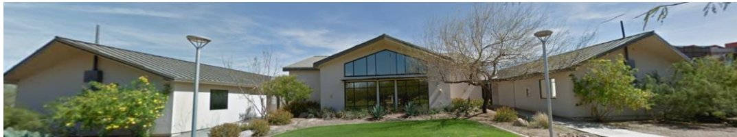
Figure 21. Sample Office Building- West Facing
