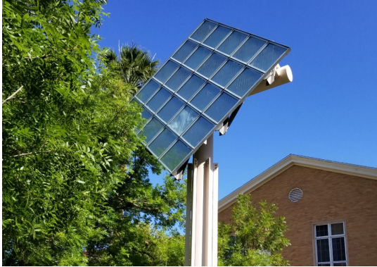
Figure 2.4: Defective Solar Panel Near Hayden Library.
