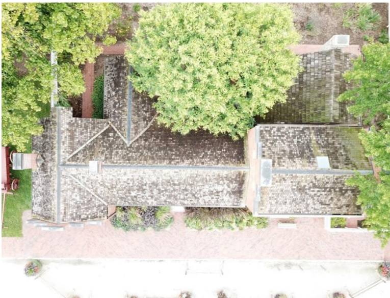
Top View of Historic Roof.
