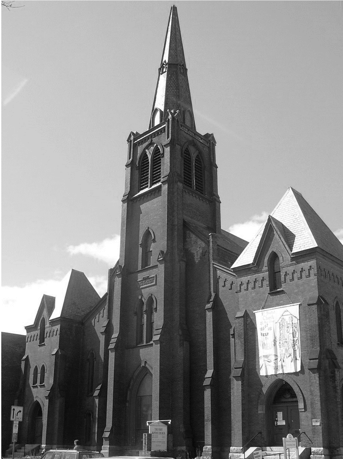
Figure 35. Photo of the Exterior of Epsilon Spires. 310
