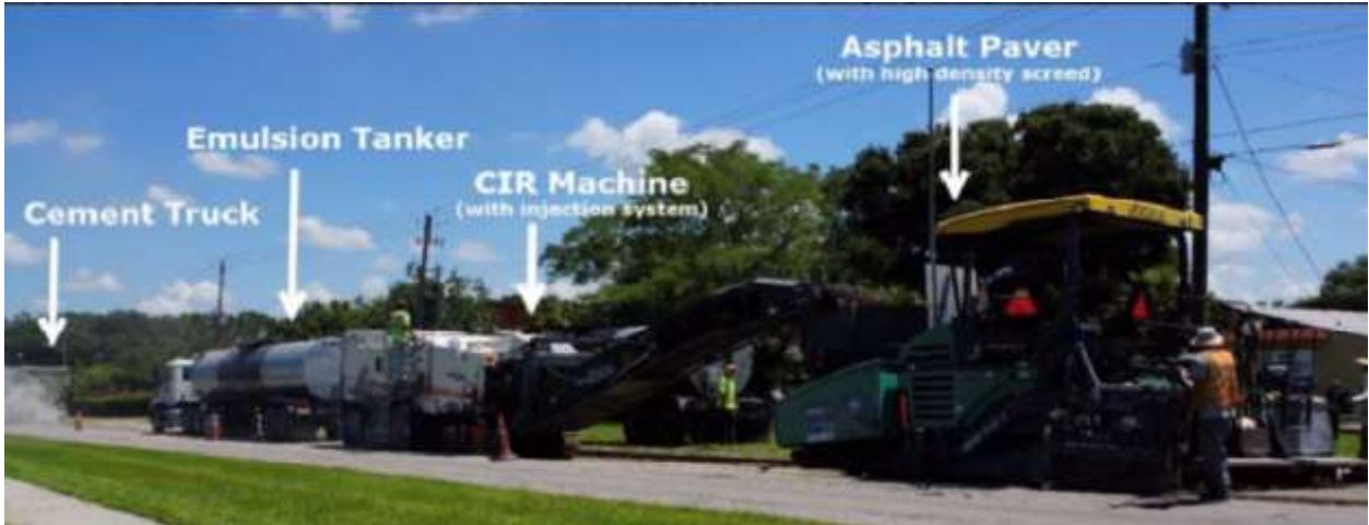
Figure 8. CIR Process (Adapted from Asphalt Paving Systems)
