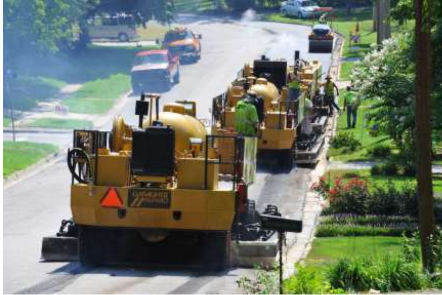
Figure 7. HIR Process (Adapted from Gallagher Asphalt Corporation, by Zeller Marketing and Design)
