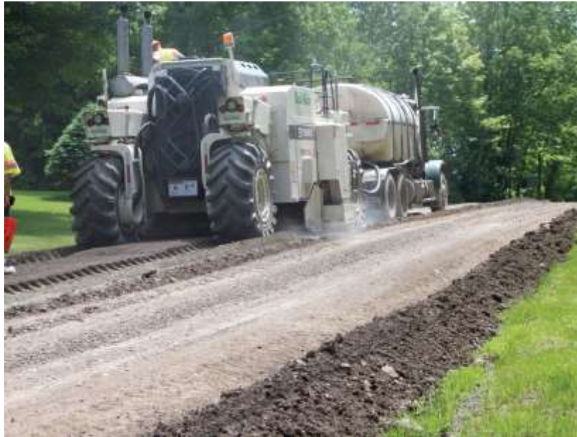
Figure 9. FDR Process (Adapted from SUIT-KOTE CORPORATION)
