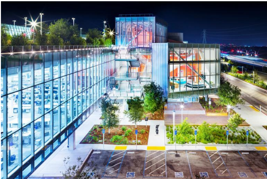
Figure 53: glass walls and skylight windows extended along the façade for natural light, adapted from wallpaper.com , by HARRIET THORPE, 2018, retrieved from https://www.wallpaper.com/architecture/frank-gehry-office-facebook-menlo-park-hq-san-francisco-opens
