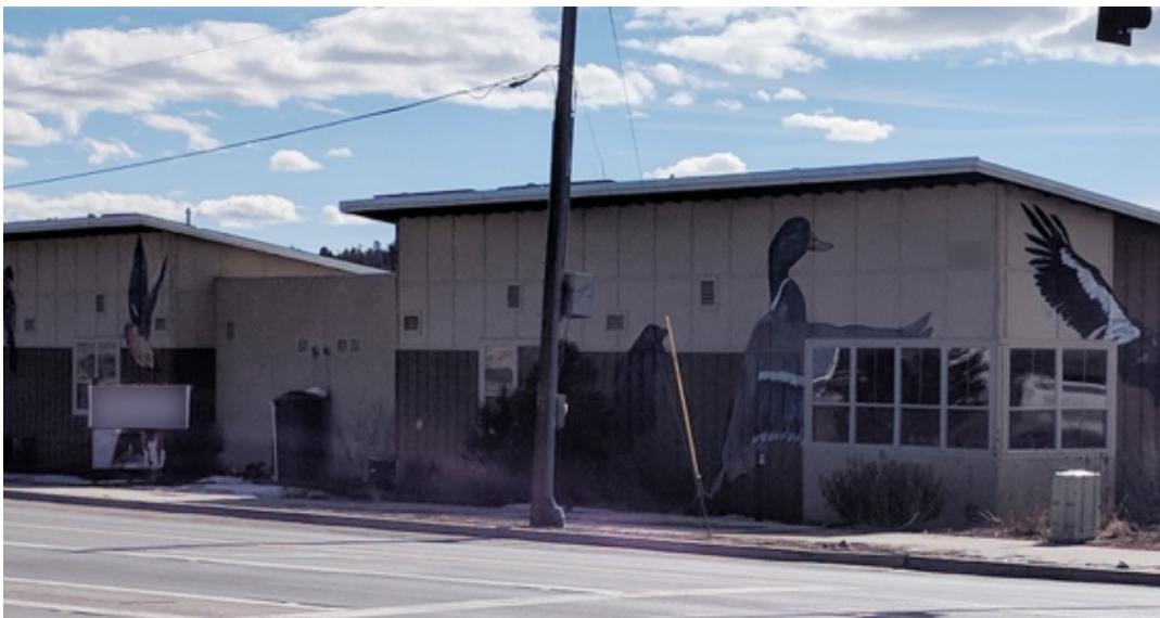
Figure 4: Photo of the school from across the street
