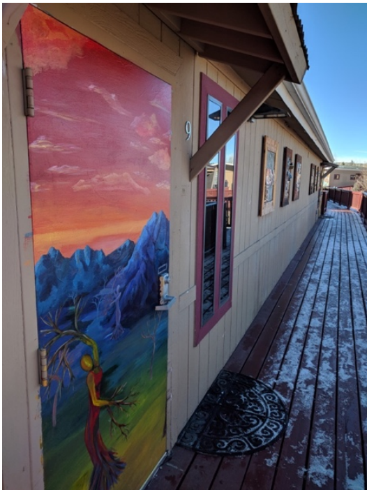
Figure 9: Photo of Deck and Painted Door
