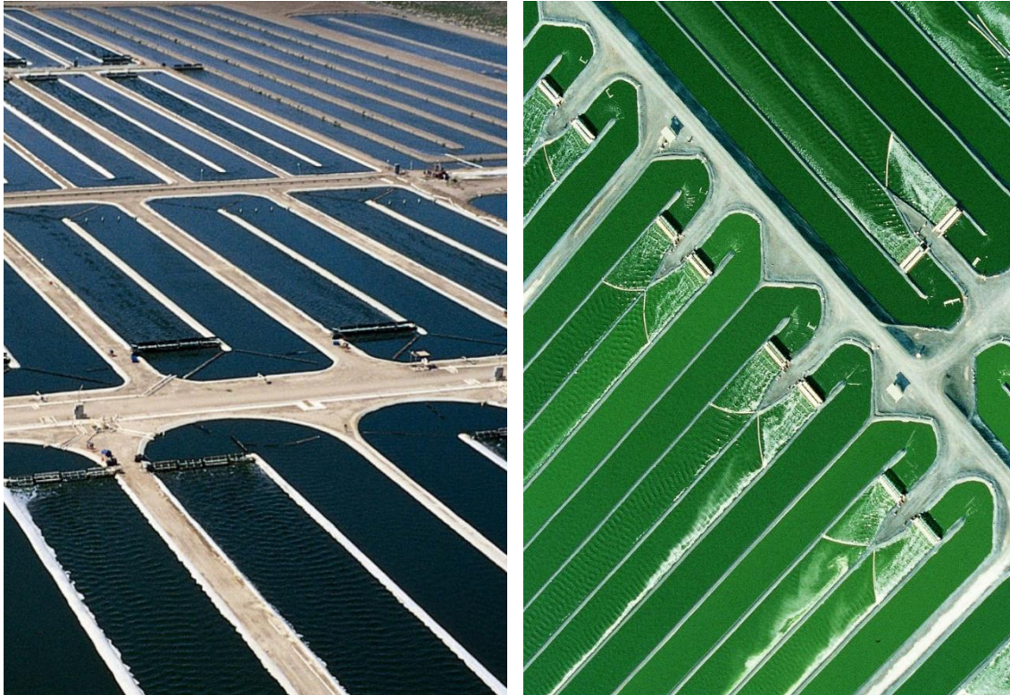
Figure 1. 4: Commercial Spirulina sp. production at Earthrise Nutritionals, LLC. in California, USA using traditional paddlewheel driven open raceways (Henrikson 2010).
