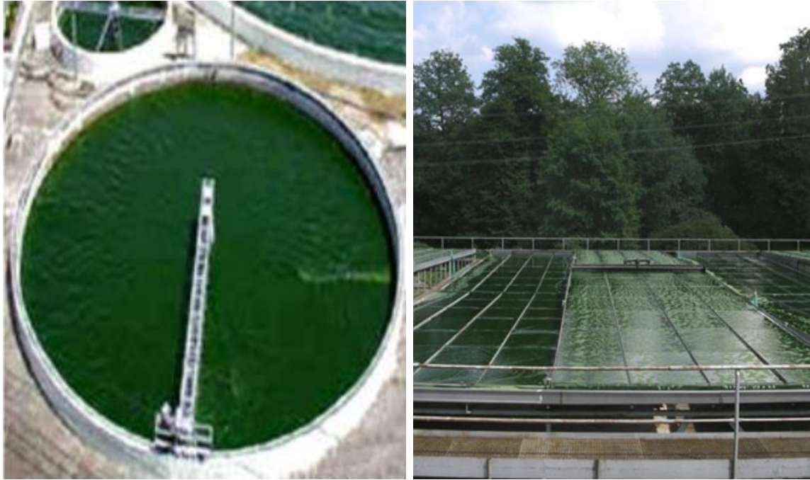
Figure 1. 6: Circular pond with center pivot mixer. Photo Credit: A. Ben-Amotz, National Institute of Oceanography, Israel.
