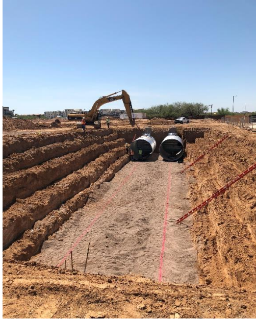
Figure 7: Construction Crew Installing the 120 in. CMP for Stormwater Storage
