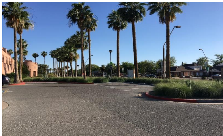
Figure 3: Permeable Pavement in Tempe, Arizona
