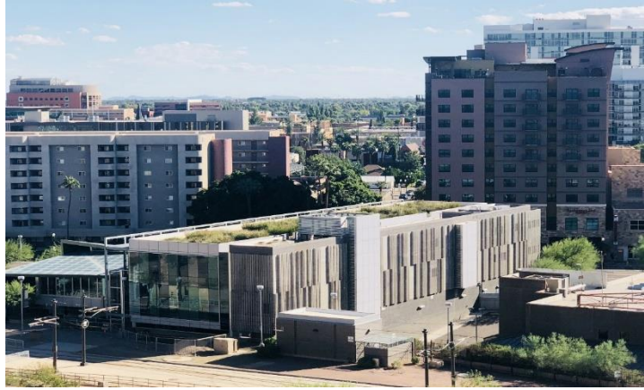
Figure 2: Green Roof in Tempe, Arizona
