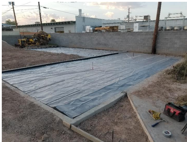
Picture 3.6: Vapor Barrier Installed on Phoenix Test Slabs
