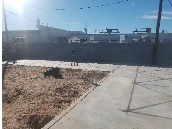
Picture 3.9: 3D Laser Scanning of Test Slabs in the Phoenix Area
