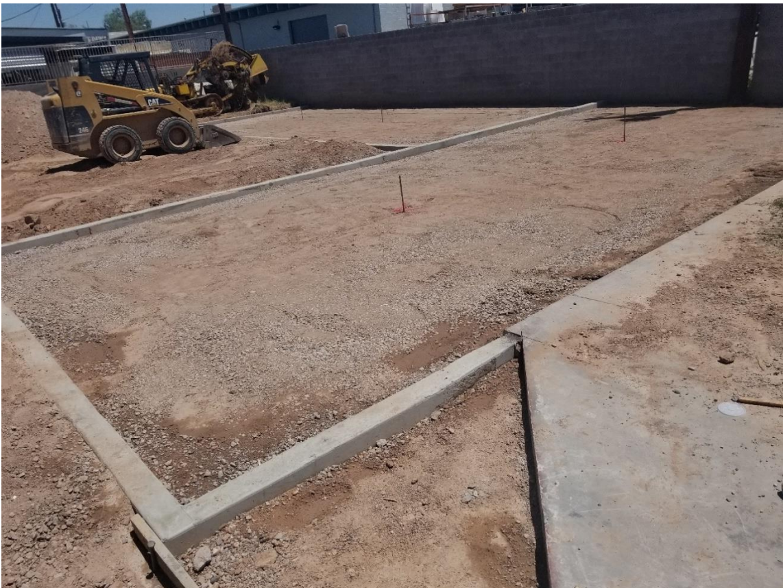
Picture 3.5: Foundation Completed and Backfilled for Phoenix Test Slabs
