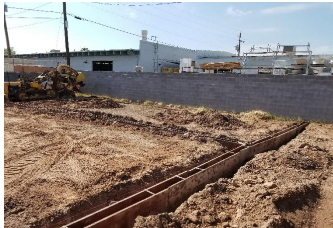
Picture 3.4: Stem Wall Forms for Phoenix Test Slabs
