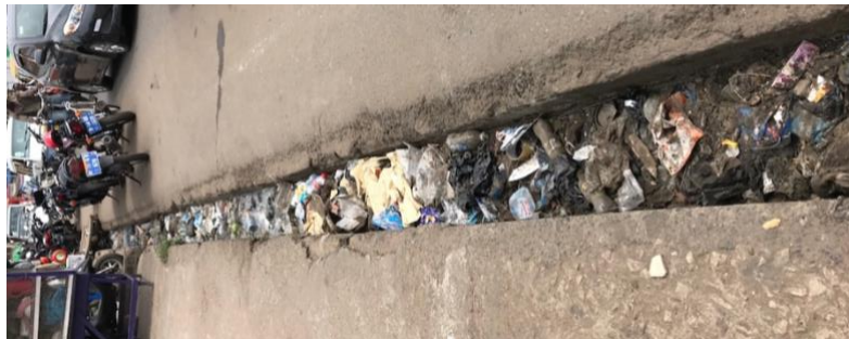
Figure 6: An open drain along New Town Road in Nima-West. Picture by Natalie Mallue 24
