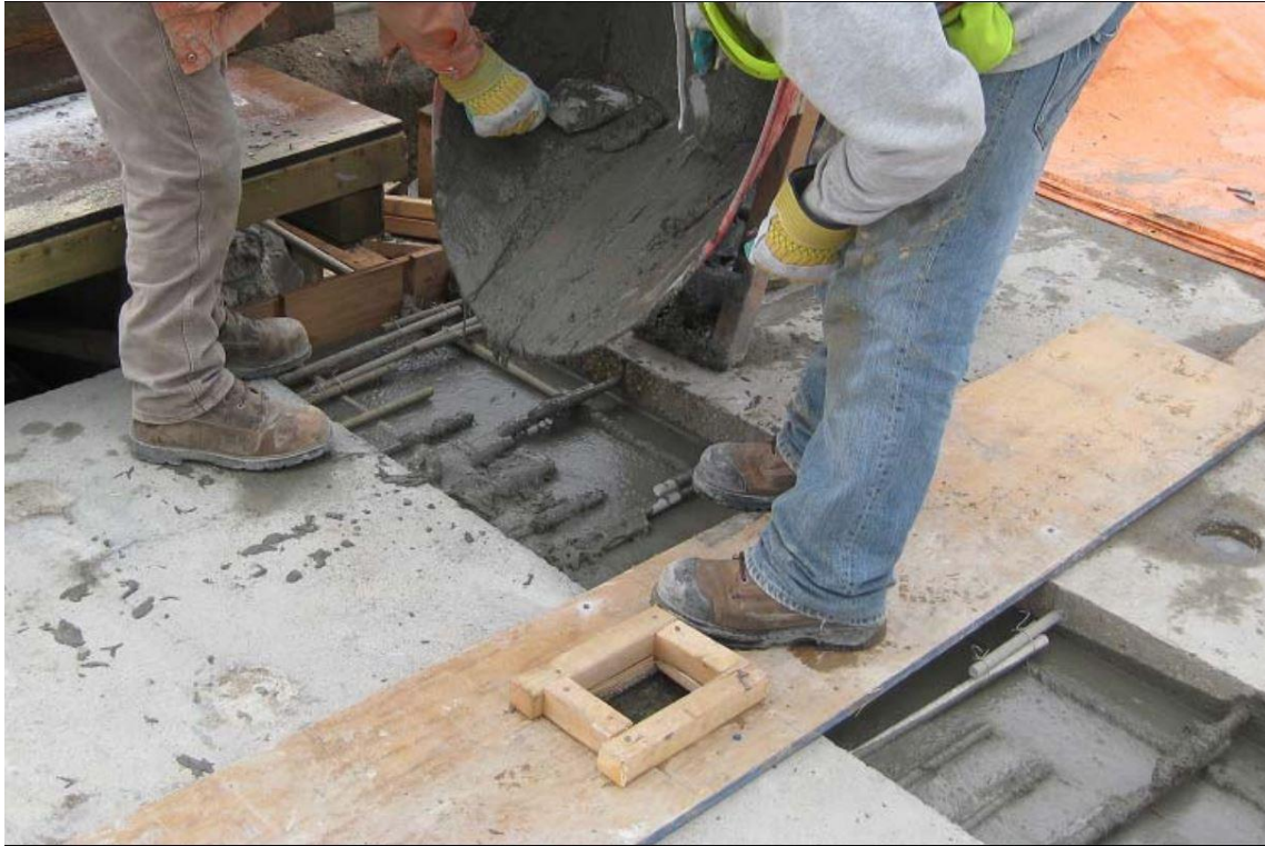
Figure 87. Filling the transverse (LLC) joints with UHPC [76].
