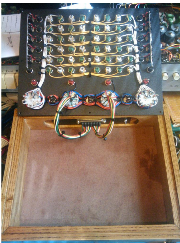
Figure 29. An image of the wiring of the “Universal Bend box.” Source: chipmusic.org/forums/topic/1121/universal-bend-box/
